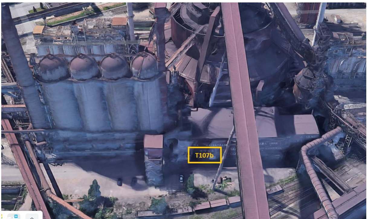
Fig. 0.4kV T107b switching station
