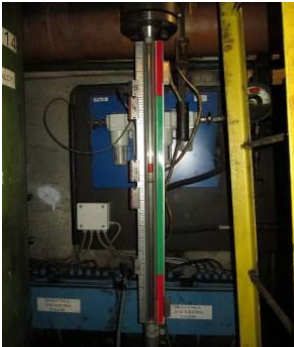
c. Optimal oil level range marked.
