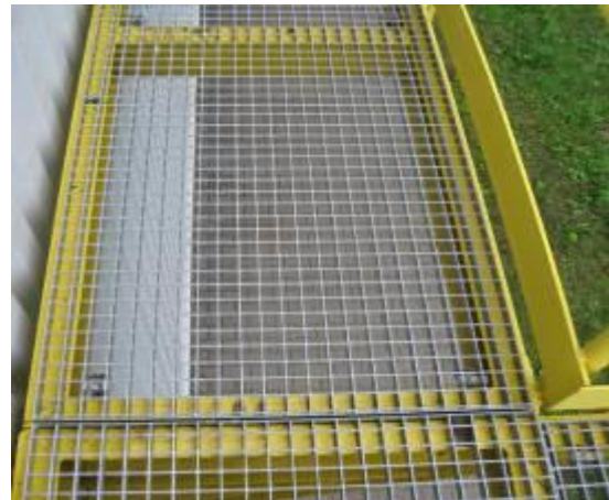
12) Platforms and covers, well fitting, adhering, secured against moving, with information about the maximum load capacity
