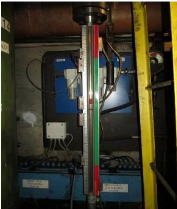
b. Optimal oil level range marked.
