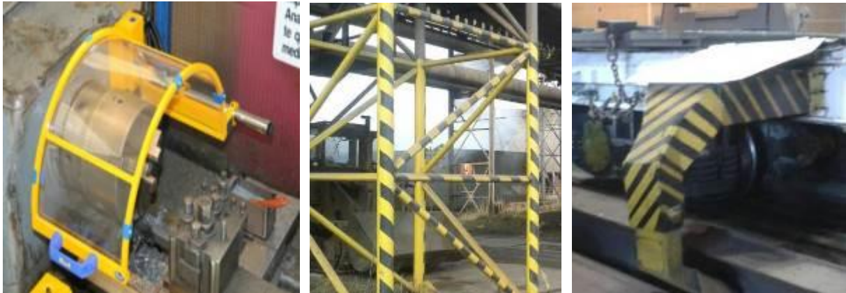
11) Railing of security zones and placement of warnings signs.
