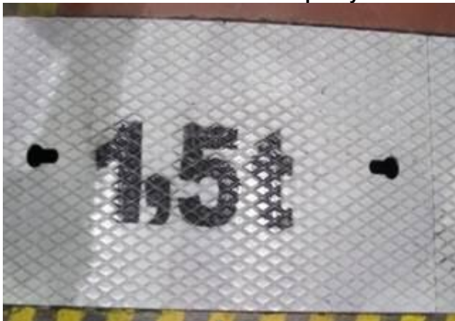
12) Platforms and covers, well fitting, adhering, secured against moving, with information about the maximum load capacity
