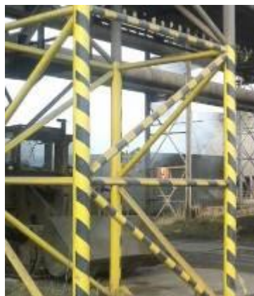
Marking of moving and protruding elements of equipment, shelter and barriers.
