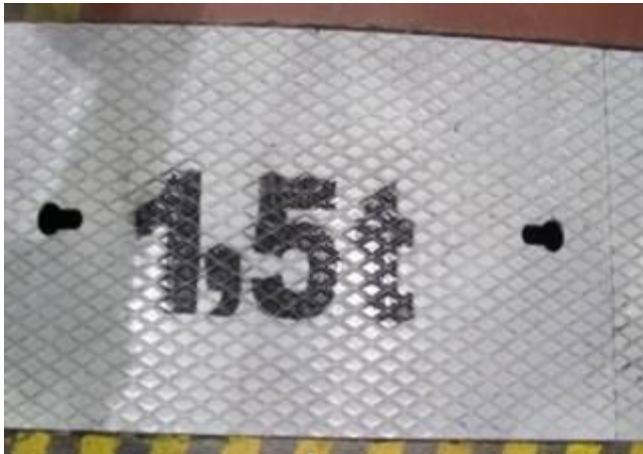
Platforms and covers, well fitting, adhering, secured against moving, with information about the maximum load capacity
