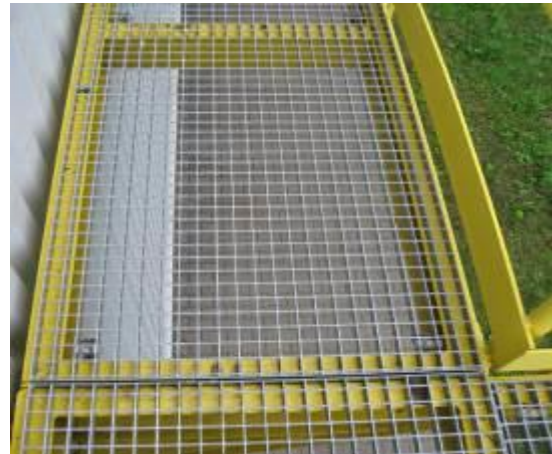
Platforms and covers, well fitting, adhering, secured against moving, with information about the maximum load capacity
